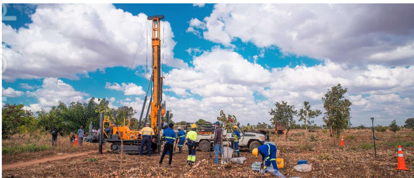
Figure 7: Core drilling at Kasiya
